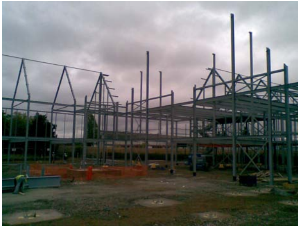
Steelwork looking towards Council Chamber area
