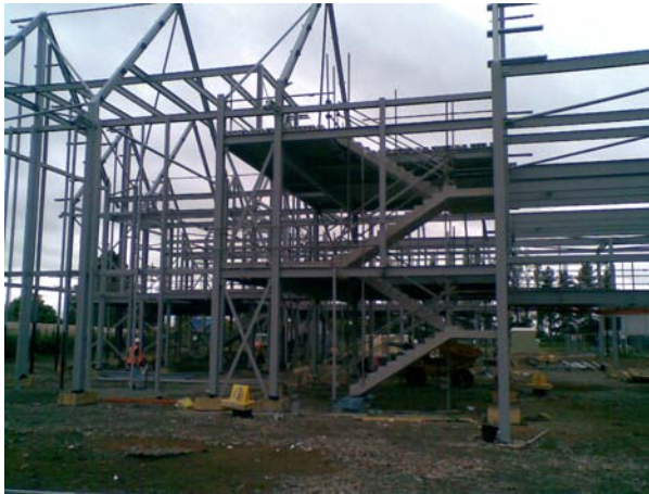
Staircase and steelwork by Council Chamber
