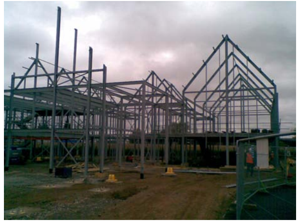
Steelwork looking towards Cafe area
