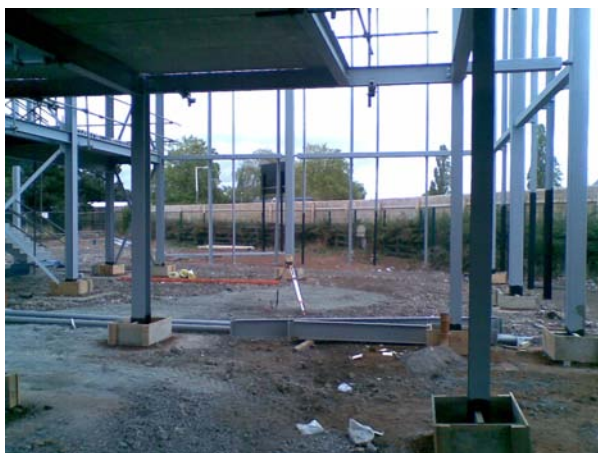
View into Council Chamber area
