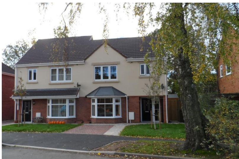
New housing at The Green, Chaddesley Corbett
