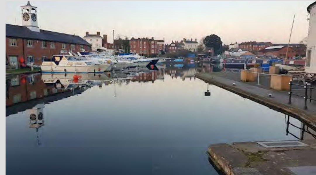
Figure 49: Stourport Basin, Stourport on Severn (Photo credit Canal and River Trust)
