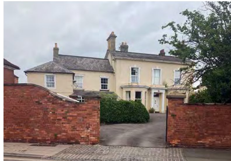
4.5.14 Oakleigh House, 17 York Street
