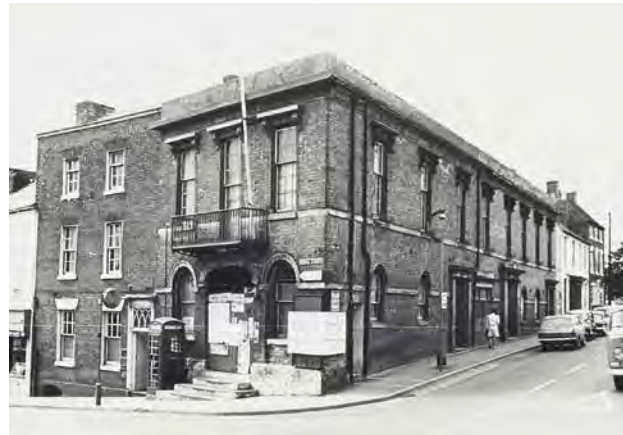
3.8 Old Town Hall, built in the 1830s, collapsed 1973 (Worcestershire County Archives and Kidderminster Shuttle)
