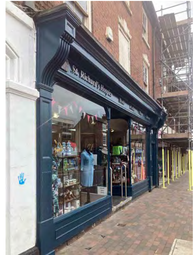
5.26 Victorian shopfront on east side of High Street
