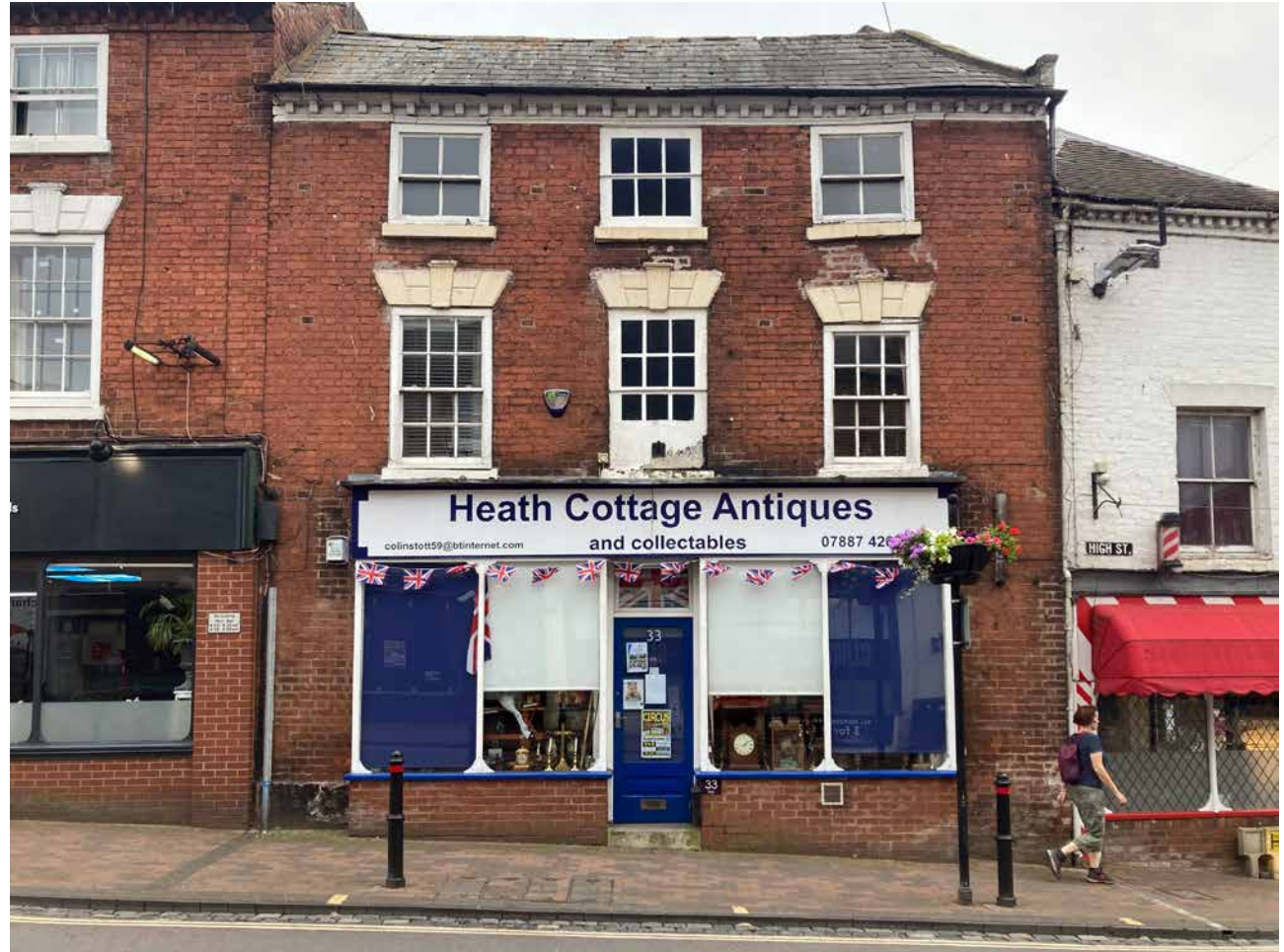
5.19 Blind windows (centre) with painted sashes. Painted brick dentil course at eaves level
