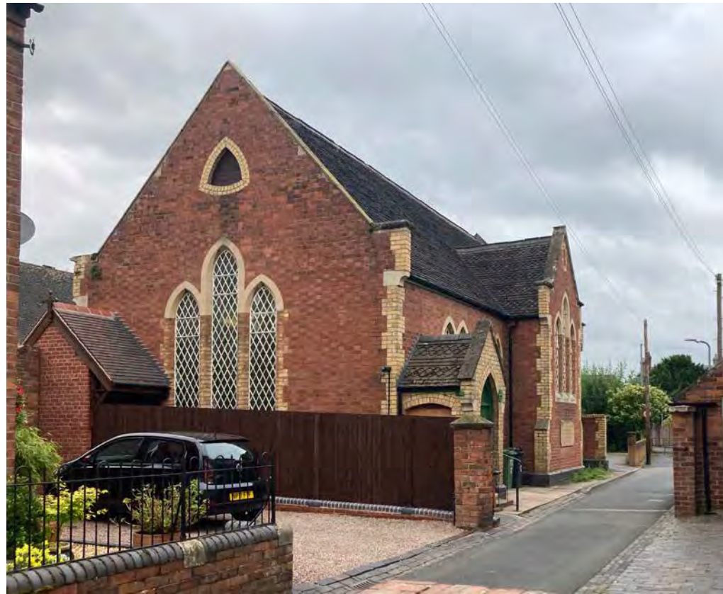
5.23 The Old School Room seen from the north
