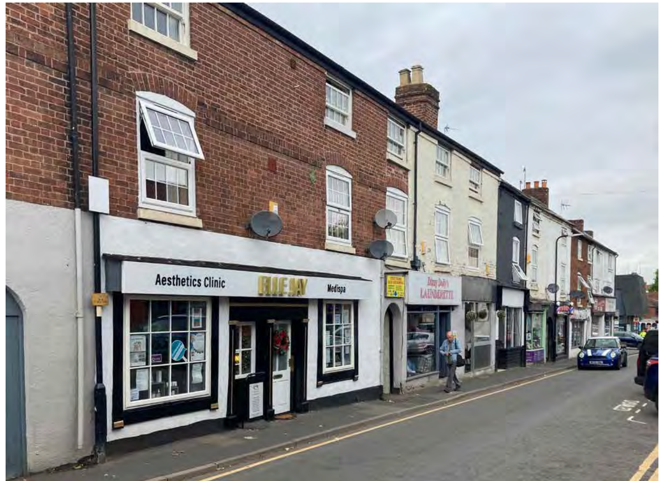
5.3 Lombard Street. Looking north at the west side
