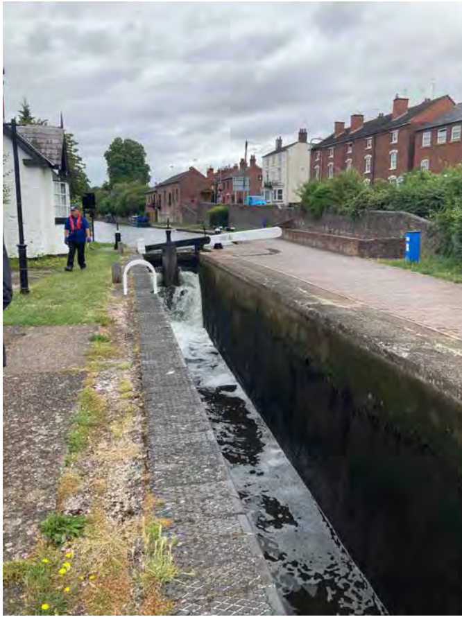
5.6 The lock north of the Wallfield Bridge at the east end of York Street
