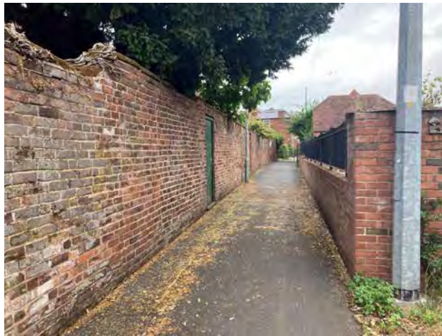
5.31 Listed wall to 17 York Street in Parkes Passage
