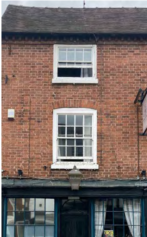
5.18 Sash windows in openings with segmental brick arches
