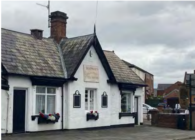
4.5.15 The Lock Shop, York Street
