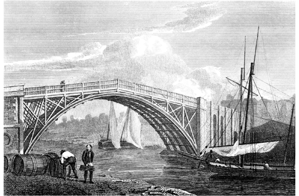
3.7 Stourport's iron bridge, built in 1806 (1812) (H68XAR (002)) (Alamy)
