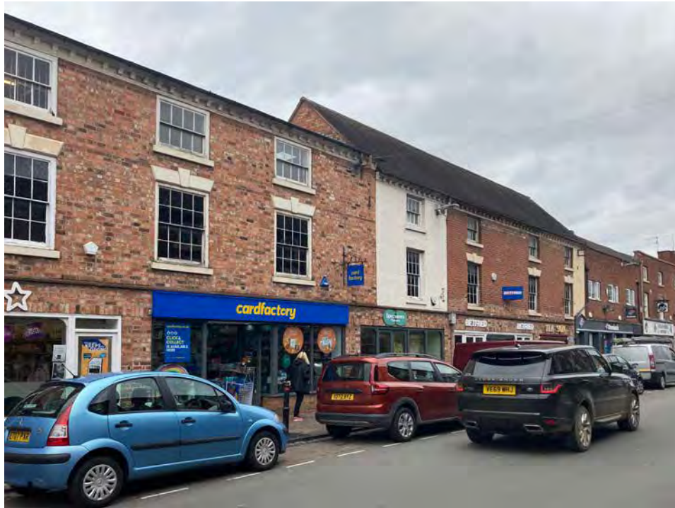
8.2 Painted brickwork detracts from the character of the building and the terrace
