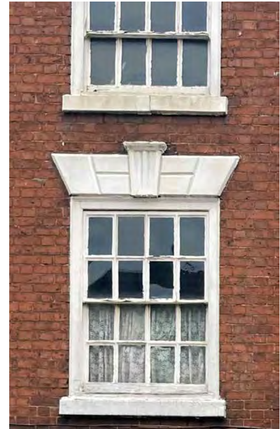
5.17 Sash windows with exposed sash boxes and voussoir arches with key stones
