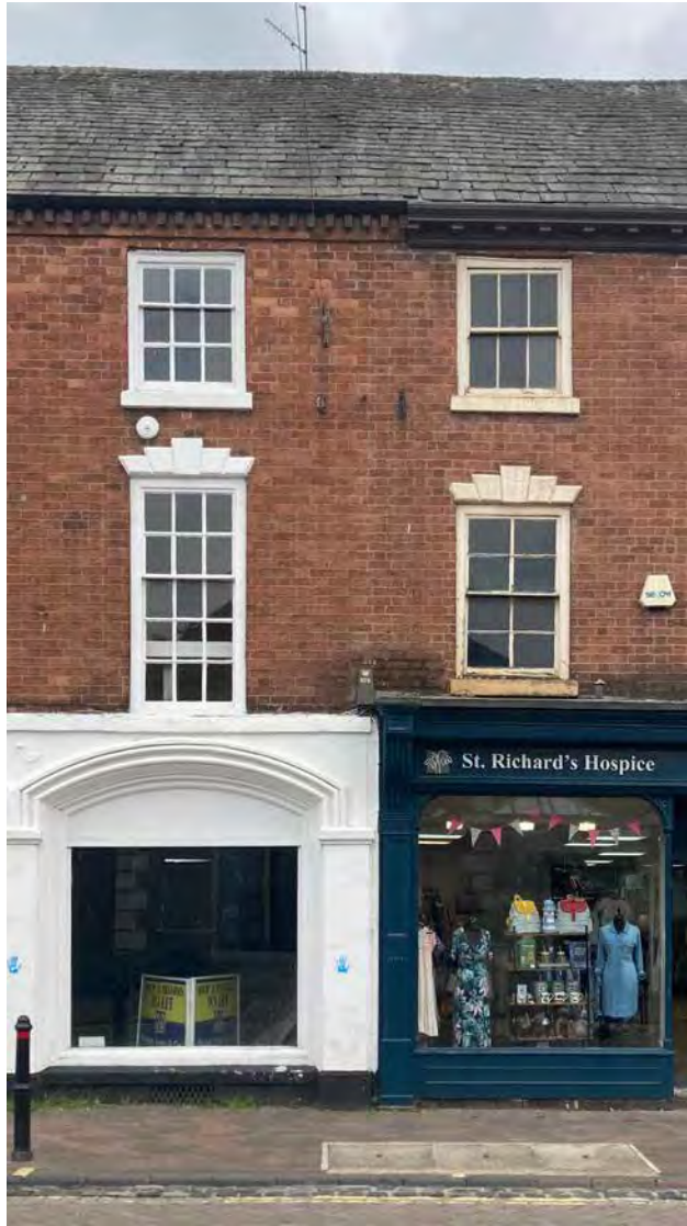
5.20 No party wall division at roof level. Note change in eaves level
