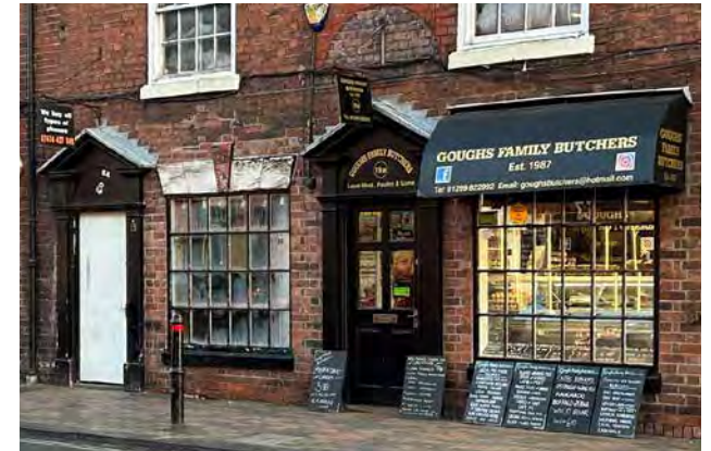
8. Nos. 19-19A High Street
