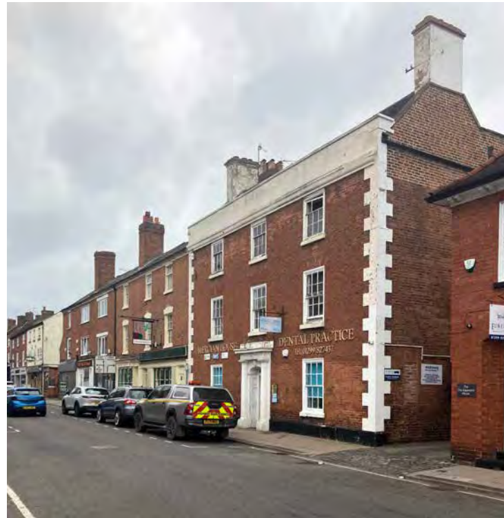
5.13 16 York Street. The largest Georgian terraced house in the CA
