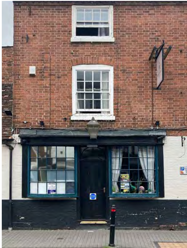
5.24 Georgian shopfront on the west side of the High Street
